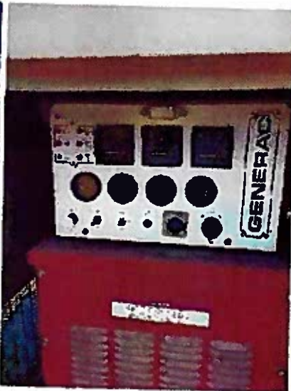
Generac 35KW Generator – Model: 89A02908-S SN:889262
