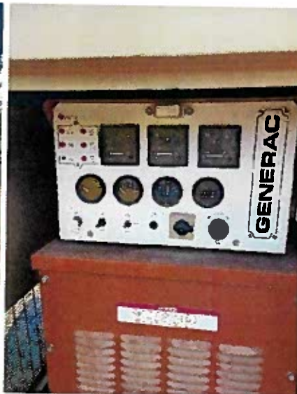
Generac 35KW Generator – Model: 89A02908-S SN:889262
