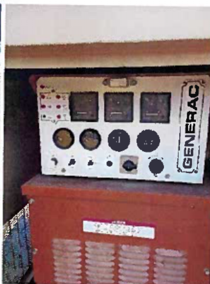
Generac 35KW Generator – Model: 89A02908-S SN:889262
