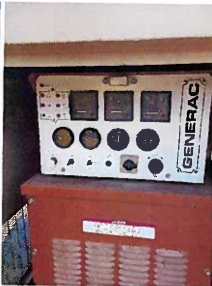
Generac 35KW Generator – Model: 89A02908-S SN:889262
